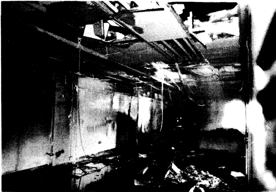
No. 65 - After extinguishment of fire for Test No. 2 looking south. Note damage to wall adjacent to planned site for Fire Test No. 3.
