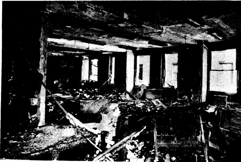
No. 47 - Another view of 7th floor fire area after extinguishment looking north and showing exterior wall. Windows seen across the open court are those of the test observation area.
