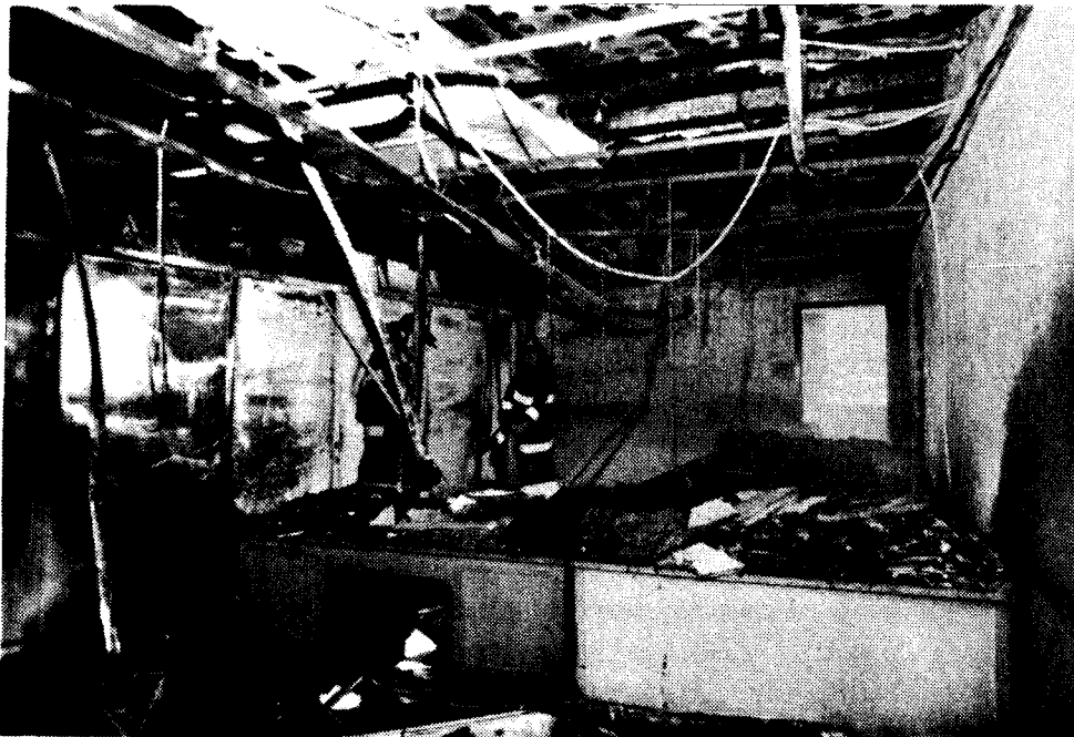
No. 64 - Final extinguishment of fire for Test No. 2. View looking towards south end of room.
