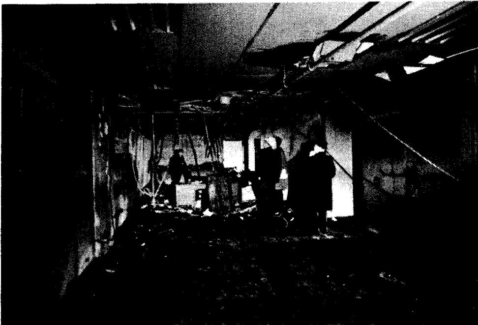
No. 80 - Area nearest the camera utilized for Fire Test No. 4 shown after extinguishment of fire for test No. 2.
