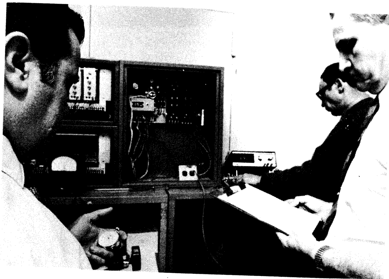
No. 30 - Recording device for smoke obscuration indicators set in 6th floor lobby area by A.D.T.
