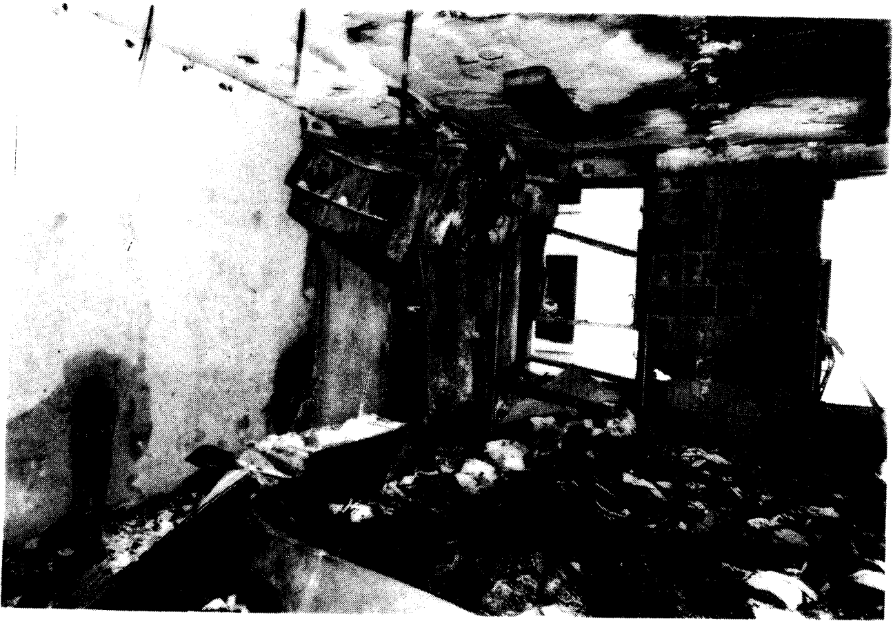
No. 48 - Close-up view north end wall Test No. 1 fire area after extinguishment showing fog nozzle openings. The two windows shown had been covered with sheet metal.
