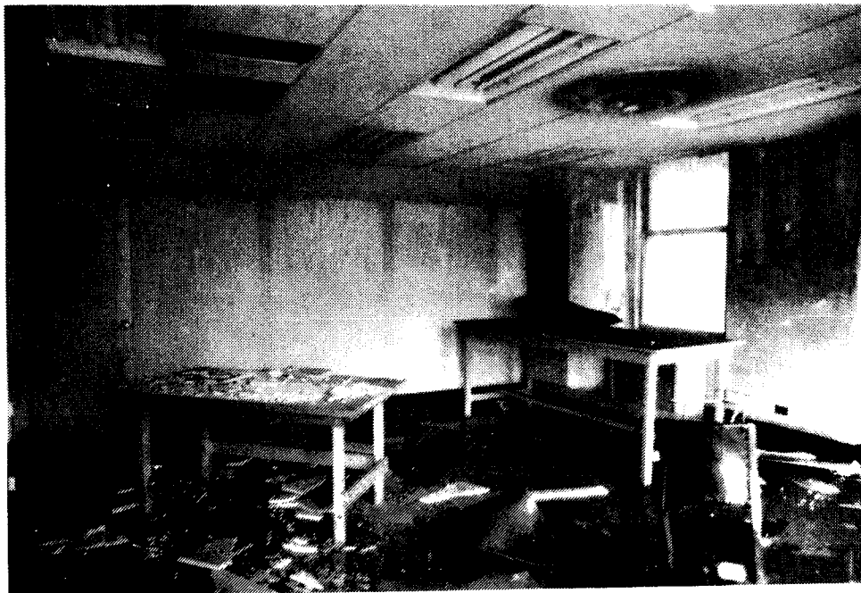
No. 77 - Fire Test No. 3 - additional evidence of the impact of the fire in another remote area at north end of 10th floor east wing.
