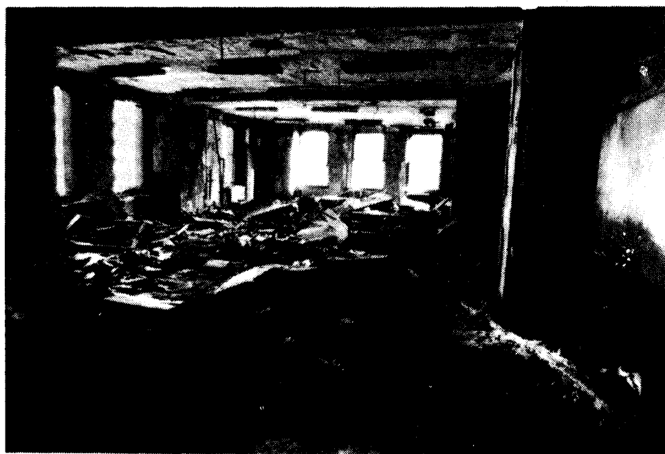
No. 44 - Test area No. 1 after extinguishment of fire. View looking south. Ceiling tiles dropped and burned. Duct work has fallen. Estimated 80 per cent contents consumed.
