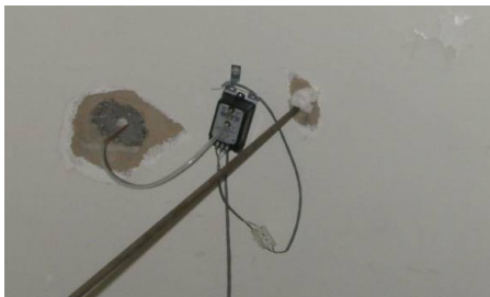
Figure 1.5-1. Pressure Transducer
