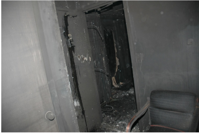
Figure 9.5-68. Into corridor from 3K apartment entrance
