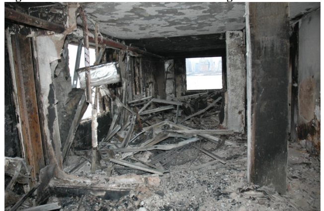
Figure 9.5-4. Through the bedrooms from the living room
