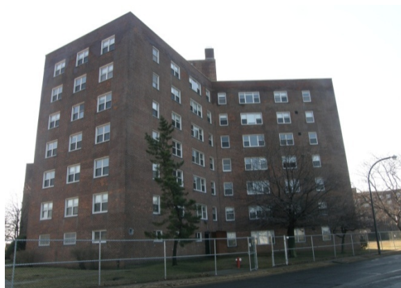
Figure 1.2-5. Right side of structure (Side D)
