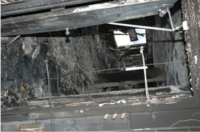
Figure 9.5-1. 7G apartment entrance
