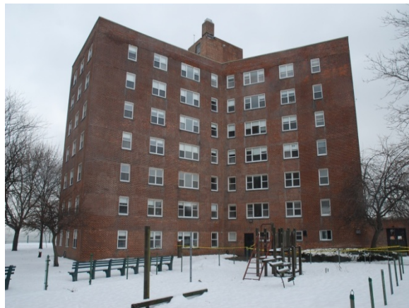
Figure 1.2-3. Left side of structure (Side B)
