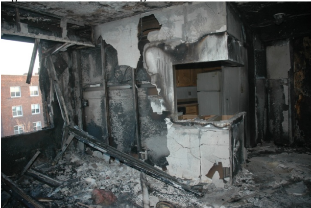
Figure 9.5-17. Living room from bedroom-side corner
