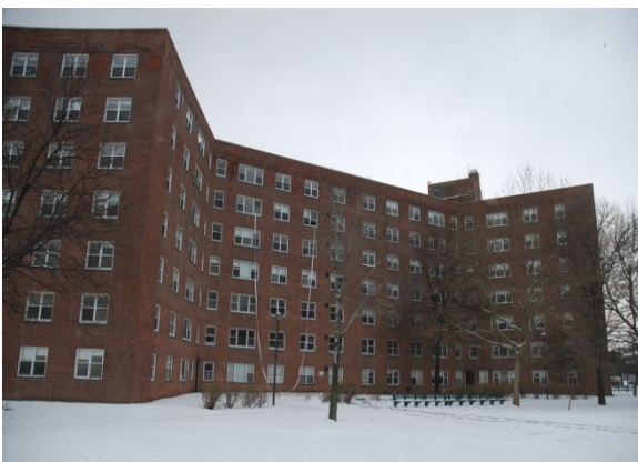
Figure 1.2-4. Rear of structure (Side C)
