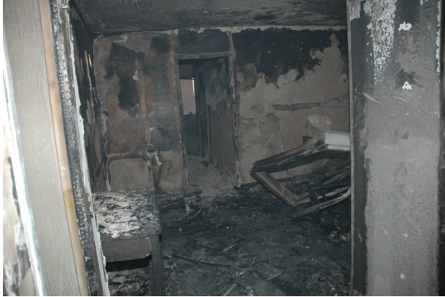
Figure 9.5-25. Living room from entrance
