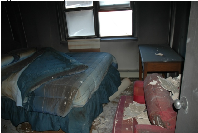
Figure 9.5-45. Bedroom 2 from hallway
