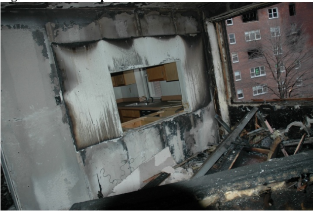
Figure 9.5-33. Living room window and kitchen
