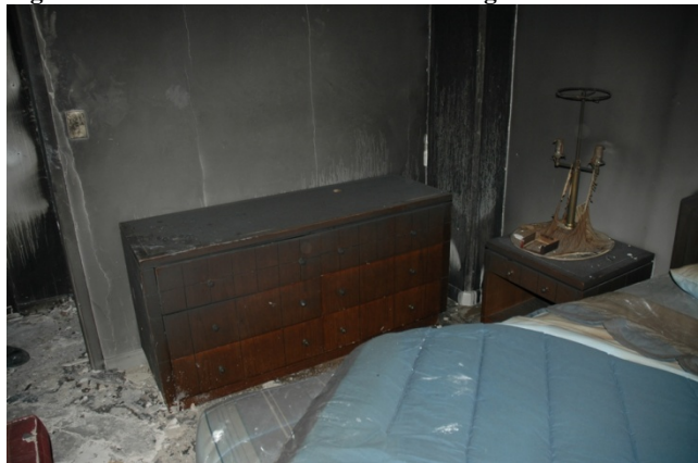
Figure 9.5-46. bedroom 2 toward hallway
