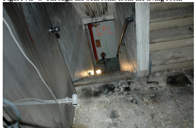
Figure 9.5-6. Down the stairwell from the fire floor
