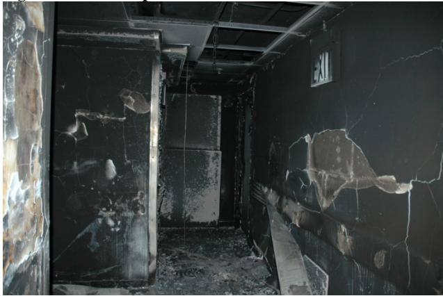
Figure 9.5-51. From apartment door into corridor
