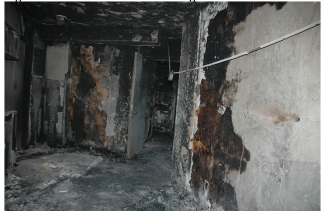
Figure 9.5-18. 7A apartment entrance from living room
