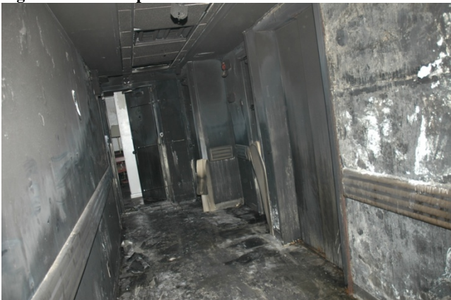
Figure 9.5-3. Down the corridor toward apartment 7K
