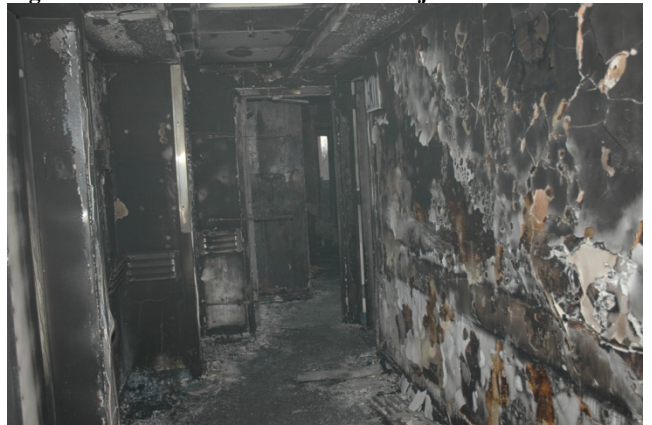
Figure 9.5-30. 5E apartment entrance from the corridor
