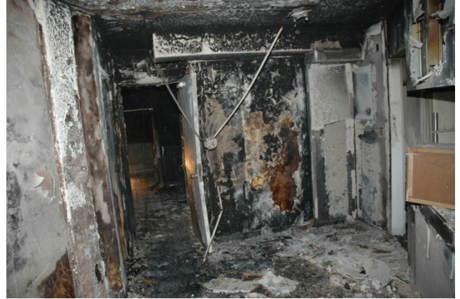
Figure 9.5-2. To the corridor from the living room
