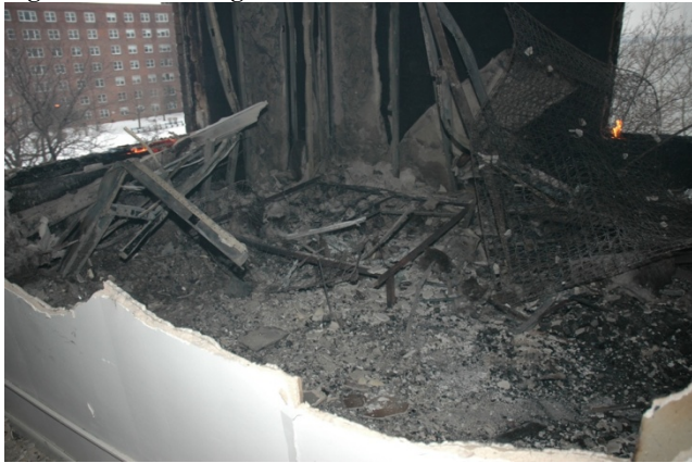
Figure 9.5-27. Bedroom windows from adjacent bedroom
